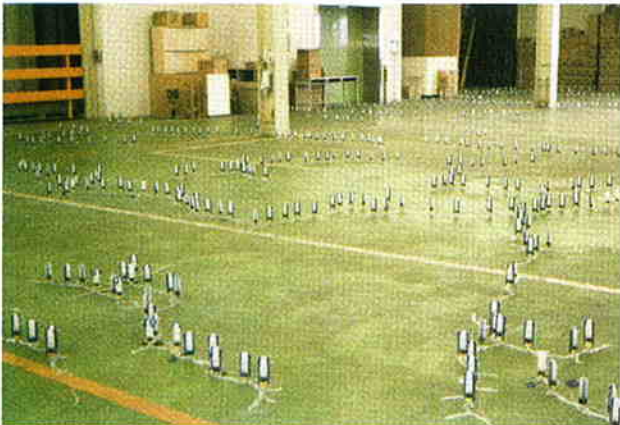
床ひび割れ補修
